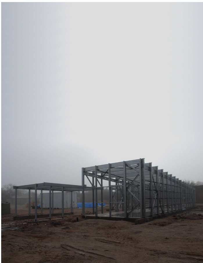
Figure 1. View of the completed ARMADILLO RESIDENCE Structural Frame. Constructed in under 12 hours, the frame, lateral, and vertical trusses are pre-fabricated components flat packed and shipped to site.
