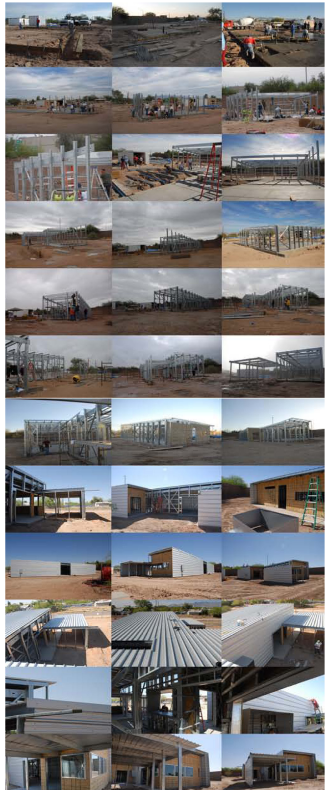
Figure 4. Evolution of the construction site illustrating the erection of the pre-fabricated frame, and introduction of other mass produced and pre-manufactured elements.
